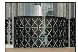
Structural system (provided with bin) elevates the holding bin for easy access and for installing handling equipment. These bin models come with one standard opening and options for up to nine openings in the x-bracing for reclaim conveyors and personnel.
