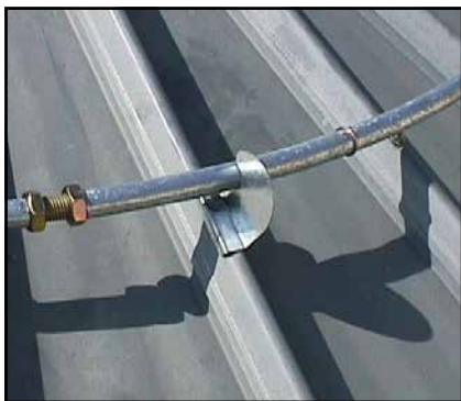
Roof Compression Rings provide additional structural support and another level of safety for those working on top of the bin.
