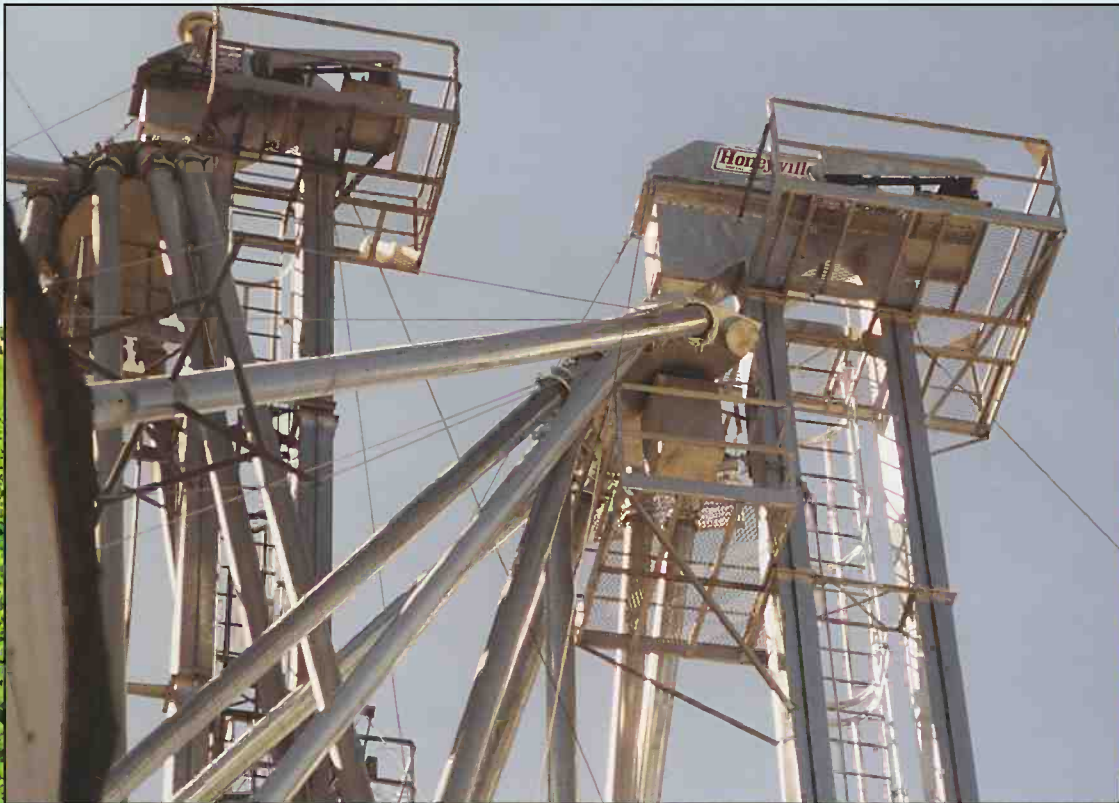
Typical installation of an EPC 8 hole distributor, shown on a model 43-24 elevator.
